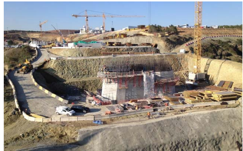
Anchorage block, side Span Piers Works
