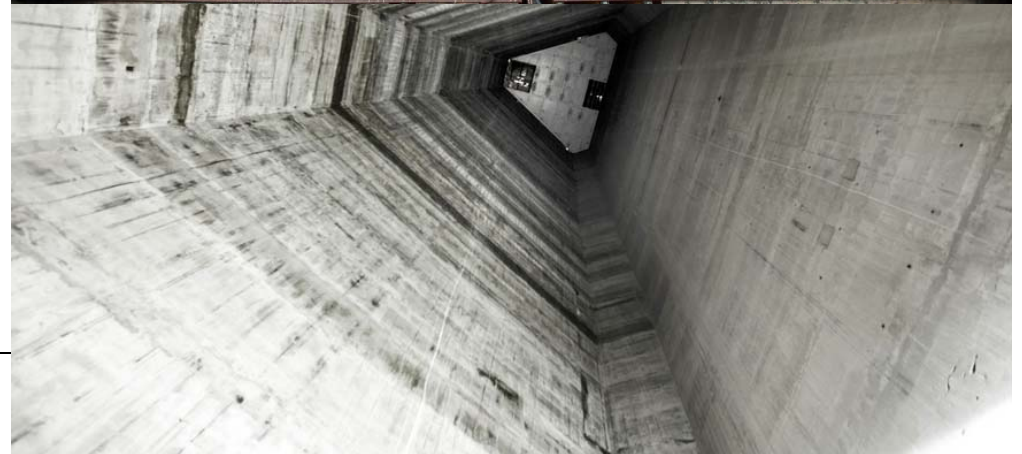
Diaphragms necessary for stiffen the zone of connection between the two legs (temporary or permanent)
