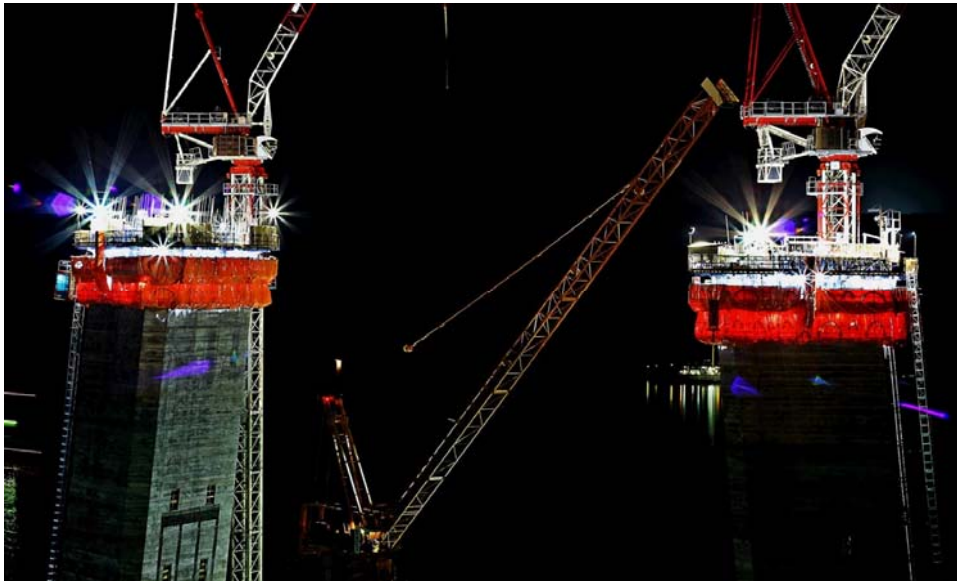
Concrete Works ongoing: nightshift
