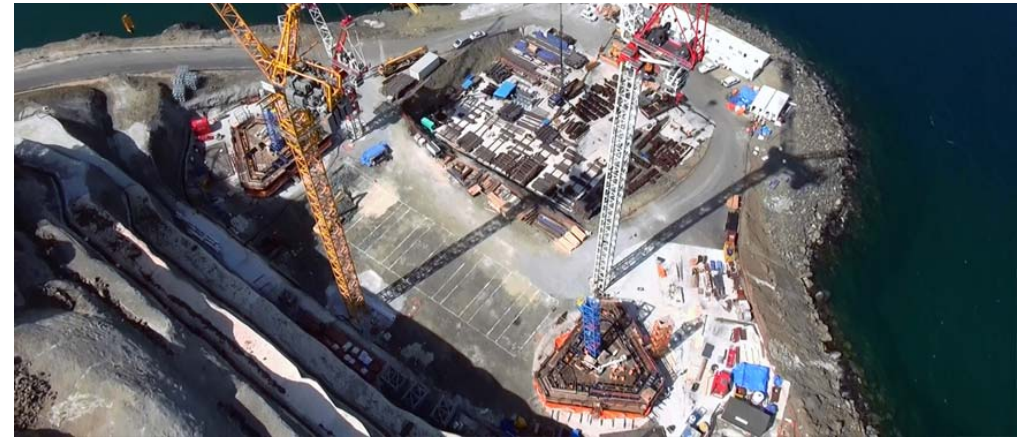
European Side – Installed Slipforms view
