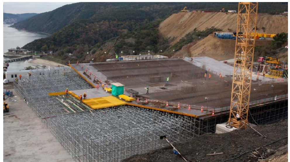
Ground Approach and Side Span Piers Works
