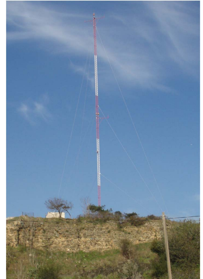
The mast installed by ICA since November 2012
